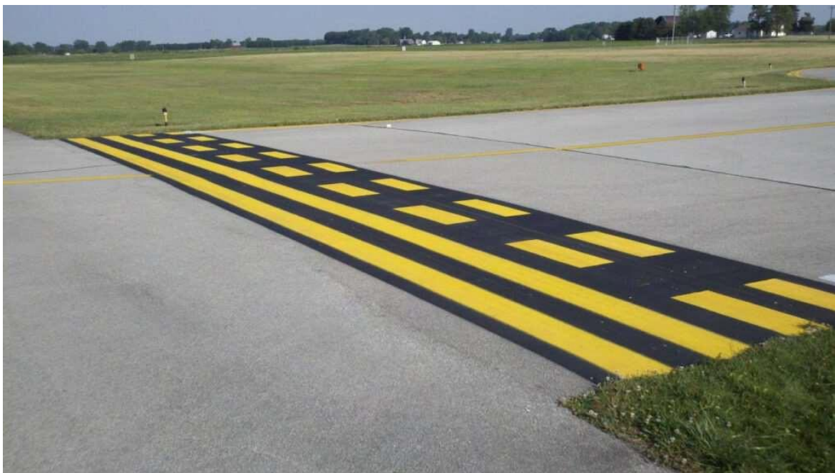
Runway holding point marking on the taxiway
