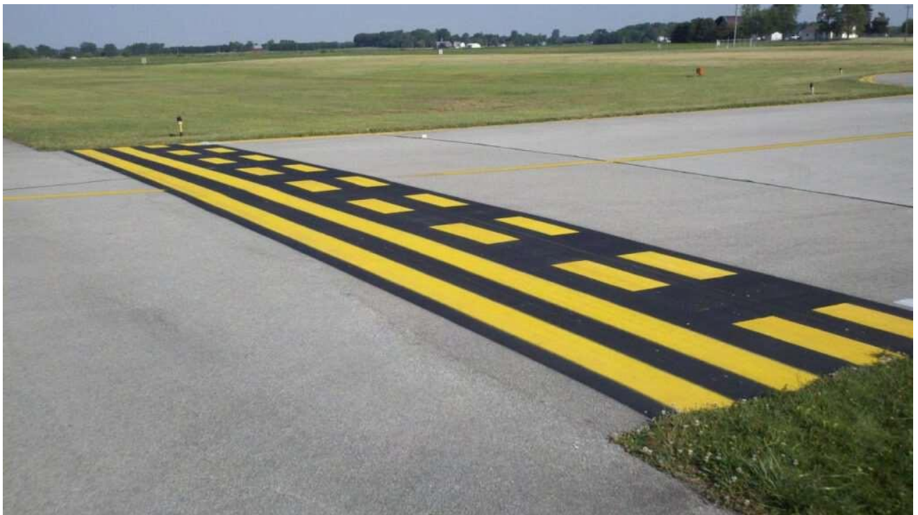
Runway holding point marking on the taxiway
